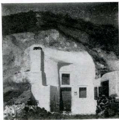
Fig. 22 —The kind of tunnels in pumice layer used for lodging, which left intact by the earthquakes of July 9, 1956. Note the field over the house.
