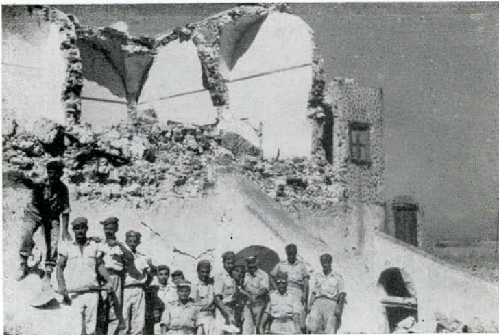
Fig. 4 —Common type of failure in Phira, Thera Island, after the earthquakes of July 9, 1956.
