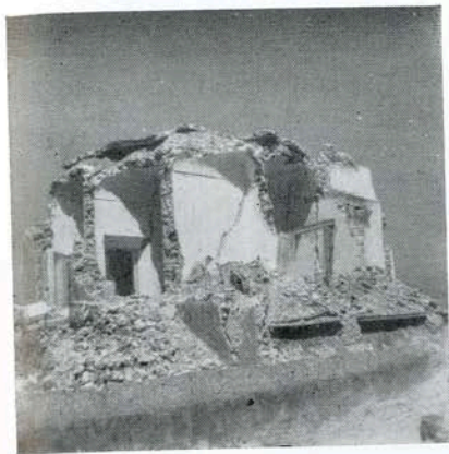
Fig. 19 —Common type of failure in Oea, after the earthquakes of July 9, 1956.
