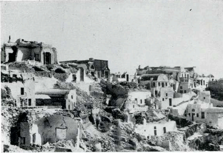
Fig. 3 —A near view showing the destruction in Phira, Thera Island, after the earthquakes of July 9, 1956.
