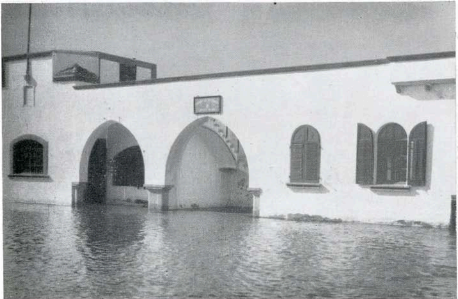
Fig. 42 —Skala, Patmos. Houses near the coast, flooded by the tsunami.
