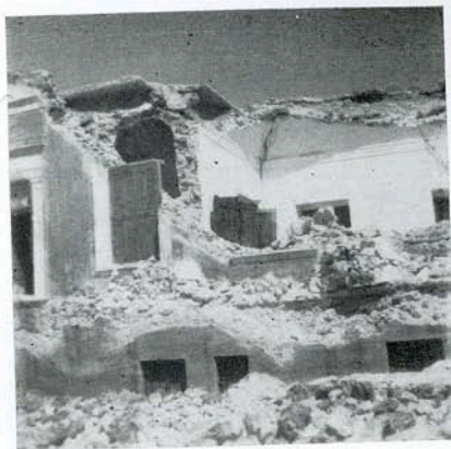
Fig. 20 —Buildings with heavy roof in Oea, after the earthquakes of July 9, 1956.
