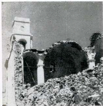
Fig. 17 —The Anastasis Church in Hemerovigli, after the earthquakes of July 9, 1956. Note that the bell tower was left intact.
